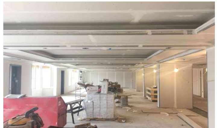
Coffered Ceiling Drywall Finishing Area G 2nd Floor
