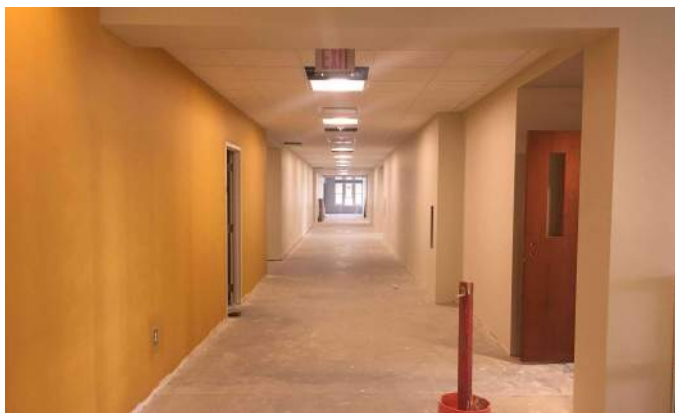
Painting Accent Walls Area A 3rd Floor
