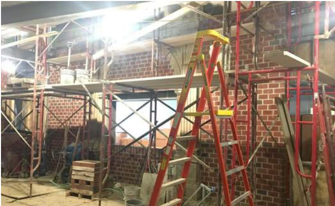
Interior Stone Veneer Installation Area F Vestibule
